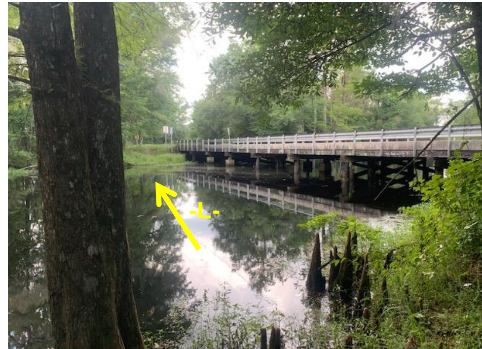
View of SR 1828 looking northwest.
